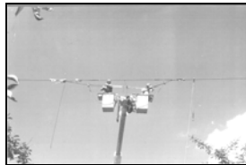
Fig. 6: Crew working from a bucket truck
