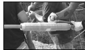
Fig. 2: Implosive splice ready for detonation
