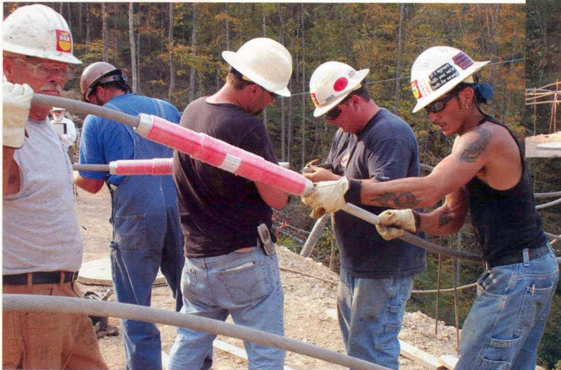
Implosive sleeves provide a low-resistance connector along with a little pyrotechnics.
